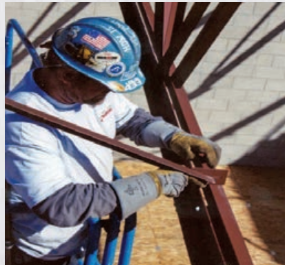
Supervisor responsibilities pertaining to open web steel joist erection.
