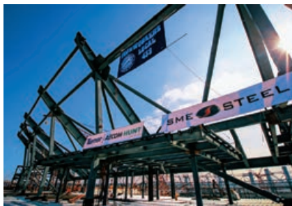
General contractors AECOM Hunt and Turner on LA Stadium.
