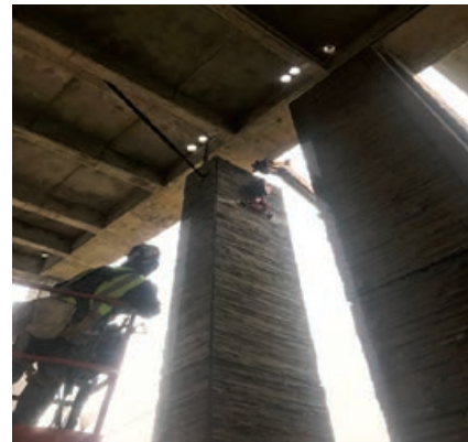
Cerner project tuck panels.
