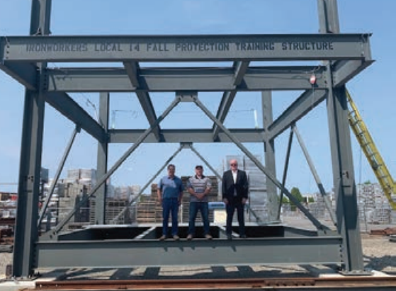
Local 14 (Spokane) fall protection training structure.
