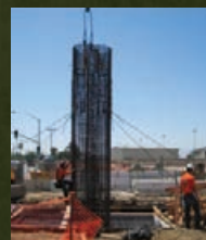
Stability requirements for vertical and horizontal columns, walls and other reinforcing activities.
