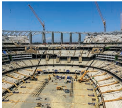
Massive stadium project utilizing teams from SME and Southwest Steel.
