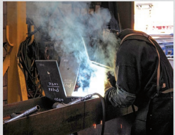
Protecting shop members during welding operations.
