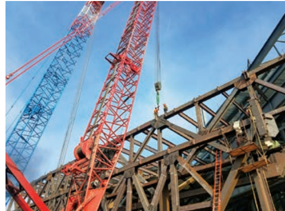
SME erects massive transfer trusses.
