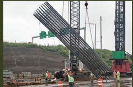
Requirements for hoisting and rigging reinforcement assemblies.
